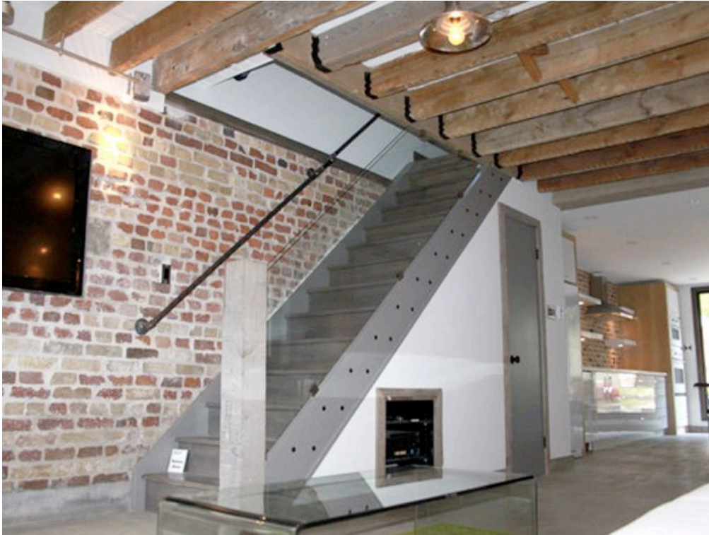
Staircase handrails of wrought iron piping are industrial in nature but look right at home on the rustic wall while the glass bordering the staircases ensures that light penetrates and the view from the living room of the exposed brick isn't compromised. Priority Management Ltd
